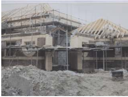
Building work still in progress
